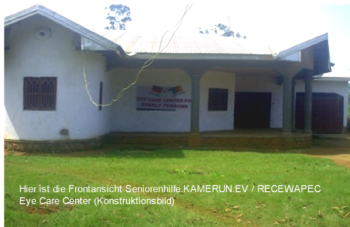
Below is the front view of SENIORENHILFE KAMERUNE.V / RECEWAPEC EYE CARE Center on construction
